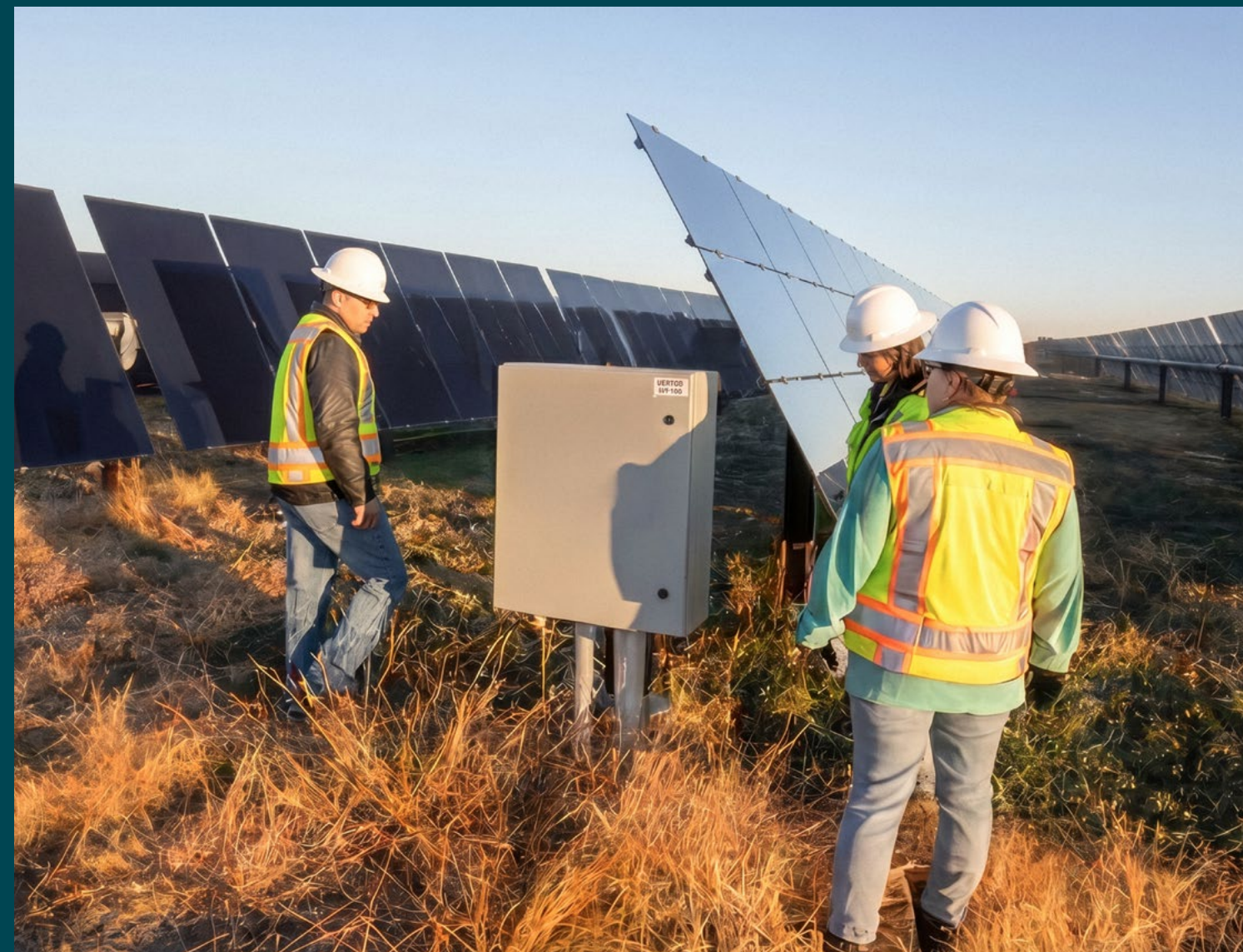
Swift Current Energy technicians at Double Black Diamond site. Source: Swift Current Energy
