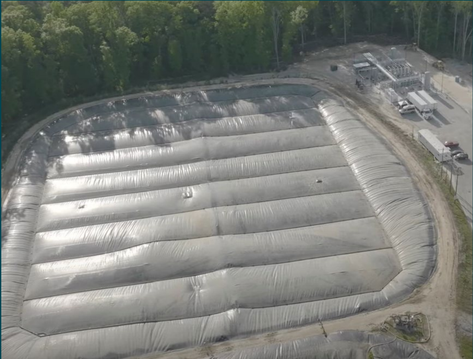
GreenGas covered anaerobic wastewater lagoon
